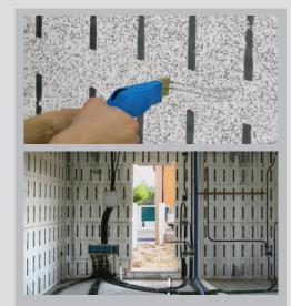
The utilities can be easily installed by the electricians or plumbers in the EPS layer, easily using a hot knife
