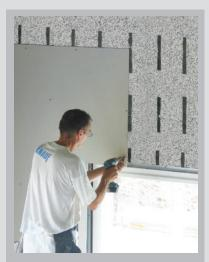
The block braces allow to fix the drywall directly on the internal wall, with no need of the aluminum structure
