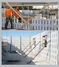
Proceed up with the layers of blocks till the required height and fix the alignment system to Climablock
