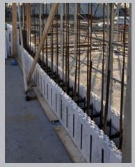
Insert the reinforce steel as per project design which will form a grid of horizontal and vertical re-bars
