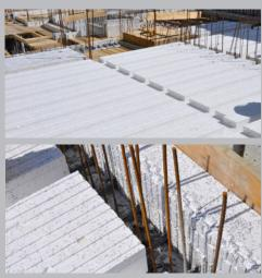
Making the raised slabs, the continuity of the external insulation is not interrupted, thus avoiding thermal bridges; moreover, the edge of the raised slabs beams is already prepared
