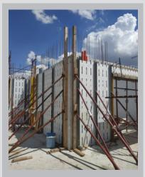
Adjust the vertical alignment before casting. Use an S4 concrete (thixotropic type, max inert grain size 20 mm)
