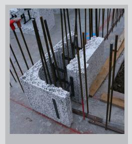
Start the first layer starting from the corners and continue with the linear blocks
